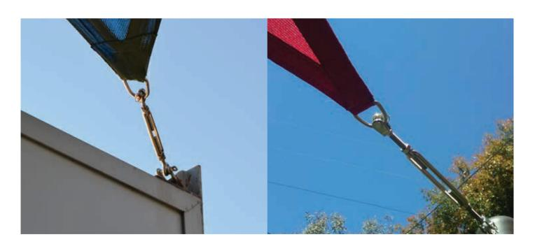
It is recommended that an anti-seize compound be used on all threaded connections to avoid "thread galling", or the binding of threads under load. This condition, though lessened, is still a possibility especially if overloaded. This is the nature of stainless steel and is not considered a defect, and Polyfab is not responsible if this occurs.
